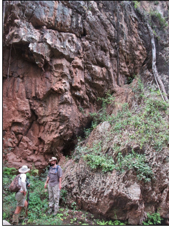
Figure 7: The crack running up the sidewall is a fault splay. Note how fractured and jointed the rocks appear near the fault.
